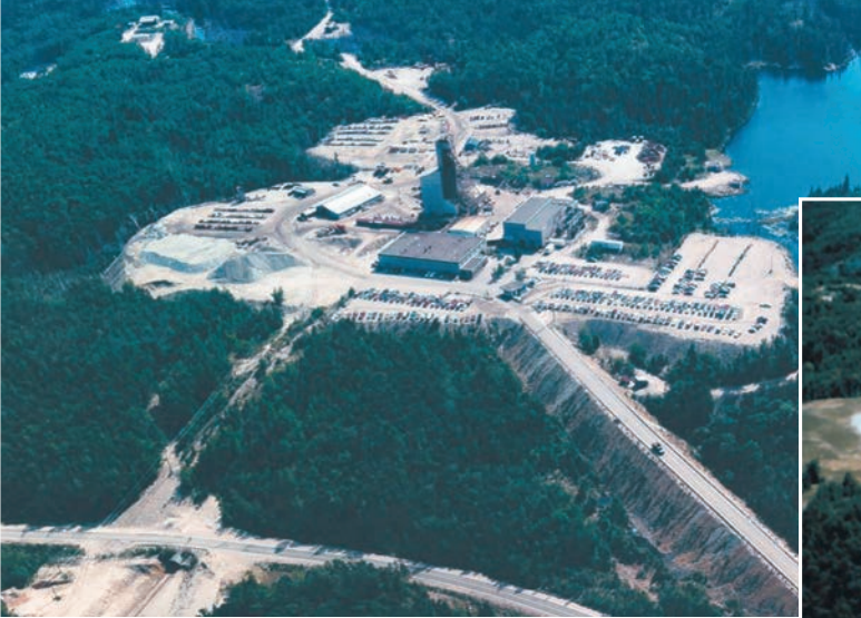
Photo of Quirke II Mine, Rio Algom Limited – Elliot Lake , Ontario prior to reclamation.
